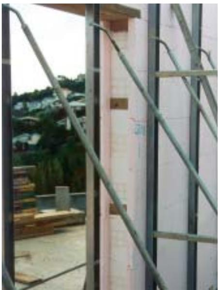
driven out of sight after bracing is removed. The adjustable arm of the brace is fastened in the same manner approximately 1300mm from the base of the wall. If under-floor heating is being installed in the concrete slab, ensure that there are no wires in this area eg: for 200mm blocks 1200 to 1400mm from the wall base.
