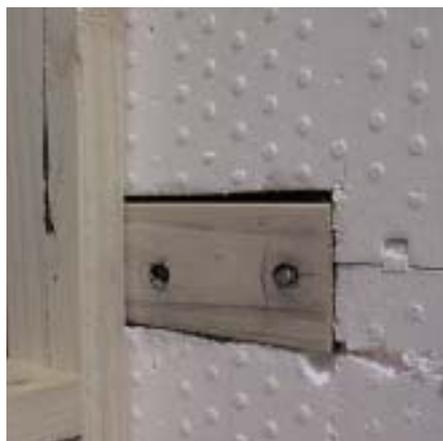
the concrete infill via cast in M12 bolts. (see Technical Manual page 78). Internal Superform BIG Block walls joining exterior Superform BIG Block walls are connected by forming a continuous concrete infill joint and providing L shaped reinforcing bars with adequate returns. A vertical reinforcing bar must be placed at the inside bend of the L bars (see Technical Manual page 77).
